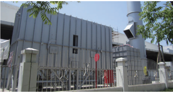
Direct-fired Regenerative Thermal Oxidizer installed in the Shanghai area
