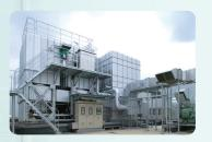
VOC treatment and odor control systems Organic solvents and malodorous gases are treated by the regenerative thermal oxidizer with high efficiency. Taikisha proposes optimum energy-saving systems combined with hydrophobic zeolite-based concentration equipment as required.
