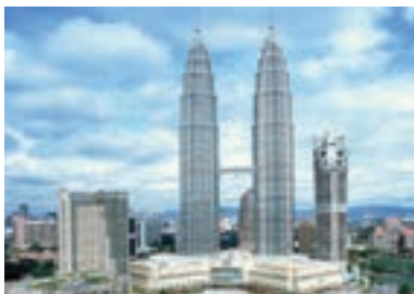
Petronas Twin Towers
