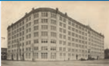
1918 Tokio Marine and Fire Insurance Building
