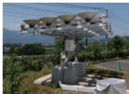
Tracking concentrator solar power generation system
